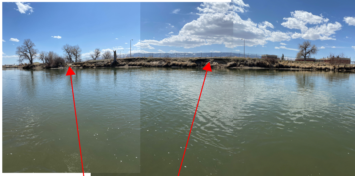
Photo 1: View south looking across the river at the unstable river bank adjacent to the Sam H. Hobbs Regional Wastewater Facility
