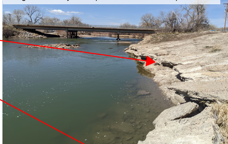
Photo 1: Layers of poured concrete visible along left bank being undercut by scour pool at least 8-10' deep.
